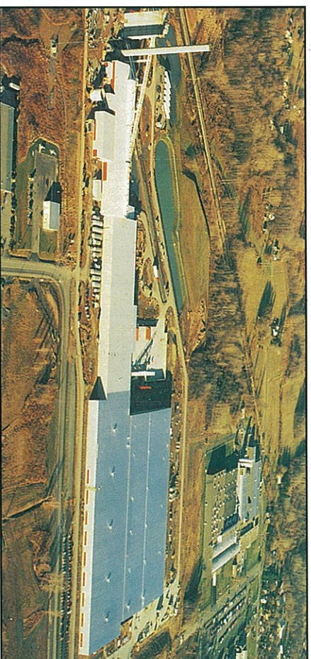
Span Construction & Engineering used pre-engineered building systems from VP Buildings for the mammoth Guardian Industries facility in Geneva, NY.
